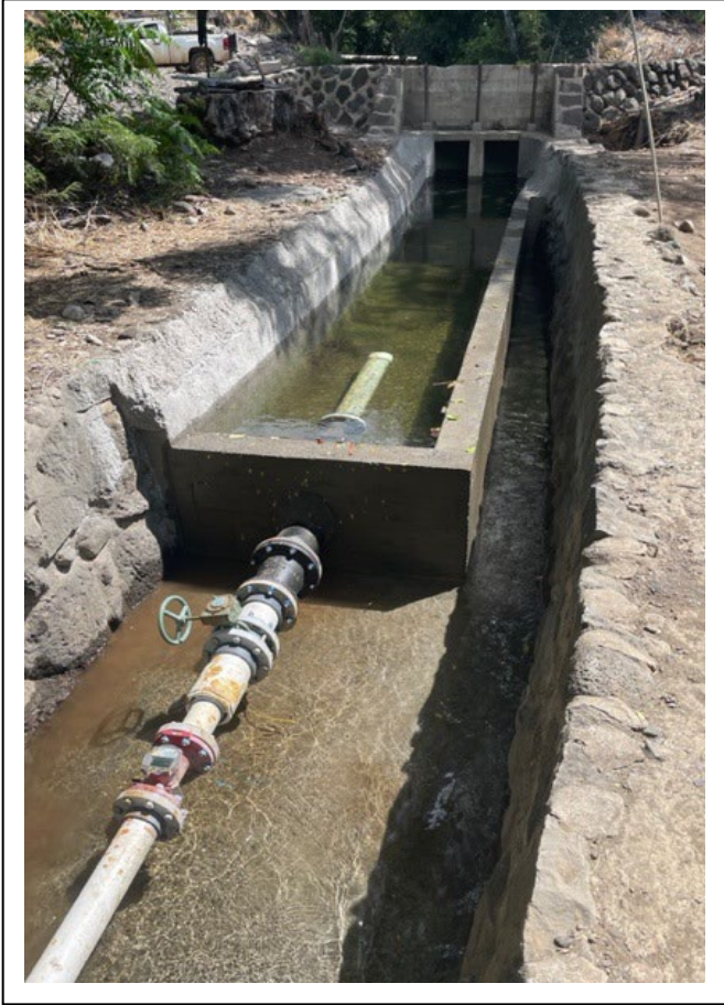
Kipuku Olowalu Intake pipe and Olowalu Weir Wall
