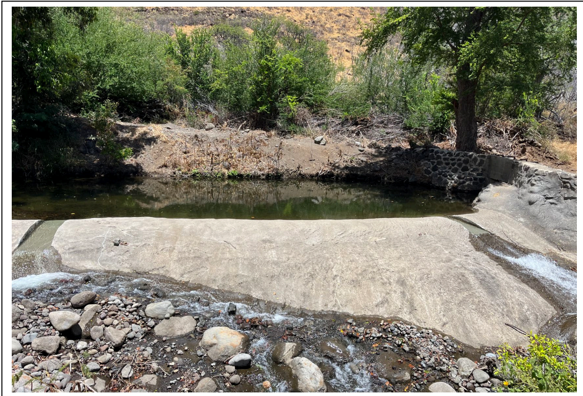
Olowalu Diversion Dam with Critter channels
